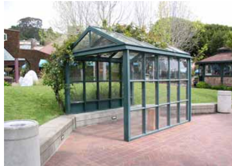
Bus shelters provide additional comfort for bus passengers, making the bus a more viable transportation option.
